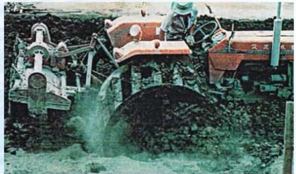
● Solidification treatment of sludge (Harbor • River • Lake)
